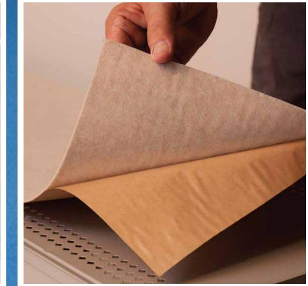
STEP 1: Peel back release paper at corners of liner
